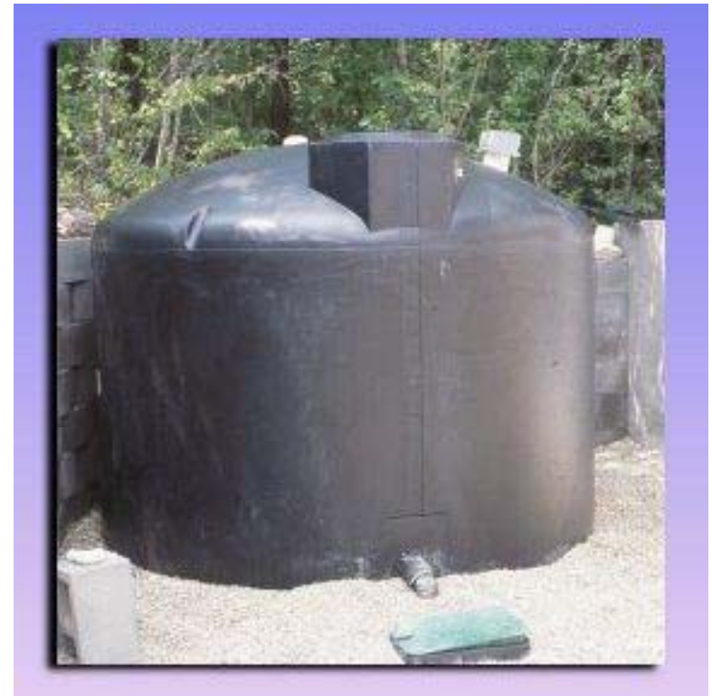
1600 gallon rain water storage tank
