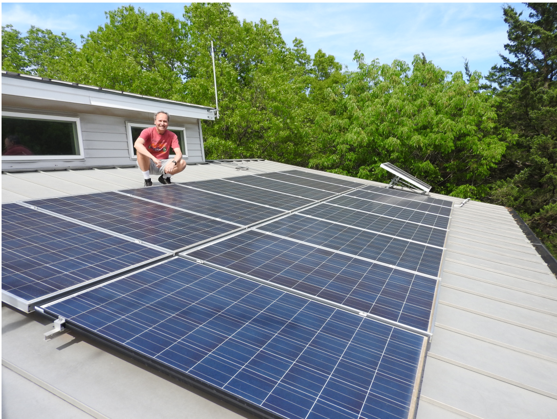
Solar PV (3.7kW) installed in 2012
