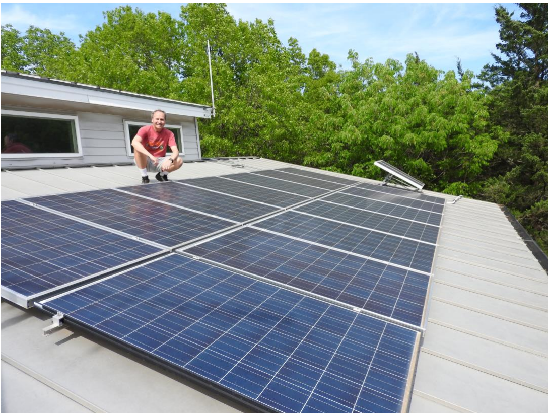
Solar PV (3.7kW) installed in 2012
